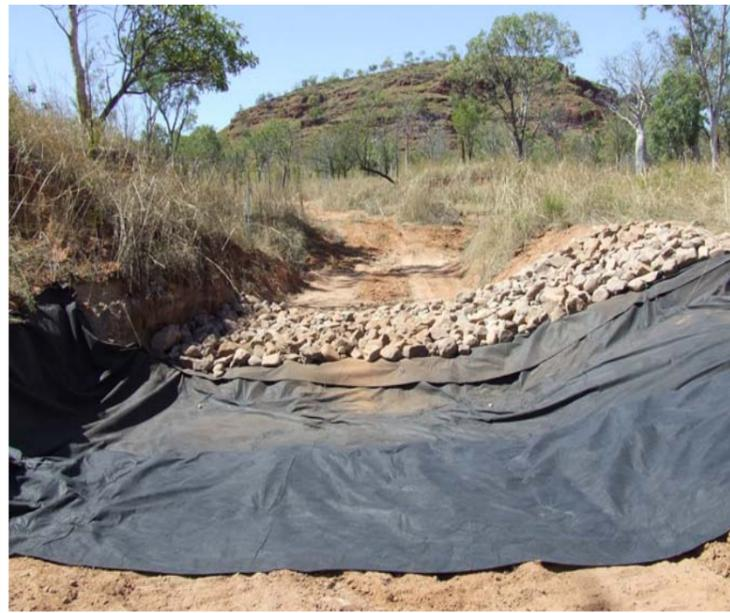
Geo textile is pinned to the bottom of the creek and covered with rocks to help slow water flows and reduce the loss of soil.
